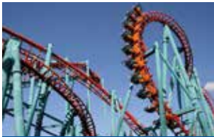
SPECIAL STEEL CONSTRUCTION
